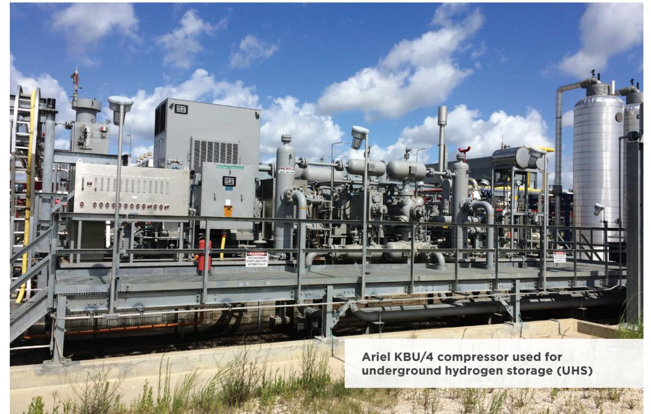
Ariel KBU/4 compressor used for underground hydrogen storage (UHS)
